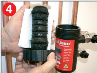
Wrap paper towelling around the build-up of sludge on the plastic sheath. Place lid assembly over a bucket and remove the plastic sheath from the magnet, remove the sludge then rinse clean. Replace the sheath over the magnet.
