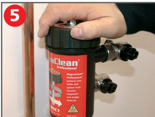
Replace the lid assembly onto the canister and close, hand tight. Be careful not to over tighten.
