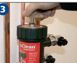
Replace the Pro-Fill air vent. Allow the system to circulate for 30 seconds. Open the Pro-Fill screw two turns and back flush until clear.
