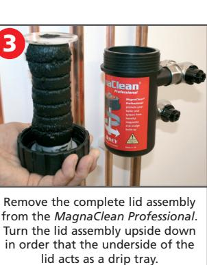
Remove the complete lid assembly from the MagnaClean Professional. Turn the lid assembly upside down in order that the underside of the lid acts as a drip tray.
