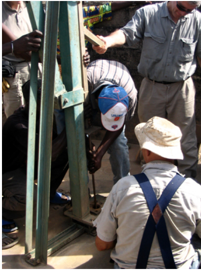
Lifewater team members coach a national in repairing a UPM hand pump.
