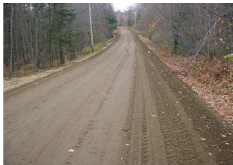
Road crowned, pot holes eliminated less sediment entering the tributary to the West Branch
