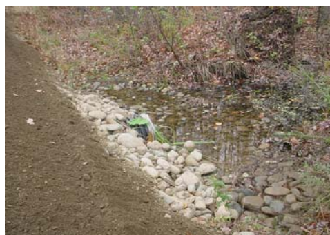
New HPPE culvert pipe. Road is not being over topped and carrying sediments in the tributary.
