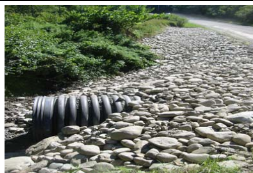
New HPPE culvert pipe and rock apron. Erosion is eliminated.
