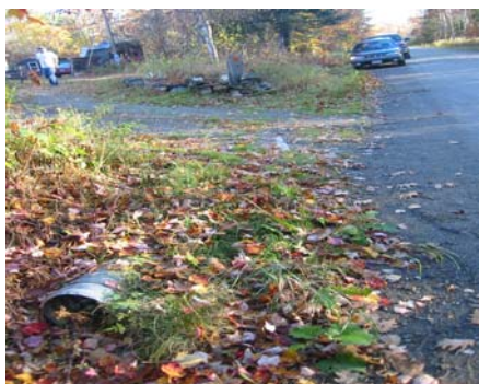
Failing culvert which leads into the tributary of the West Branch on Marden Hill Road. The culvert is blocked and sediment is carried over the culvert in a rain event.
