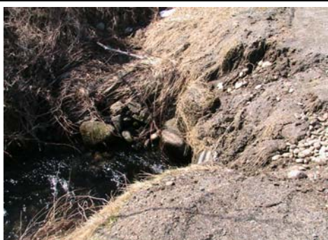
Large failing culvert which leads into the tributary of the West Branch on Marden Hill Road. The culvert is blocked and sediment is carried over the culvert in a rain event. Also no armored apron is present to take channelized flows from the roadway.
