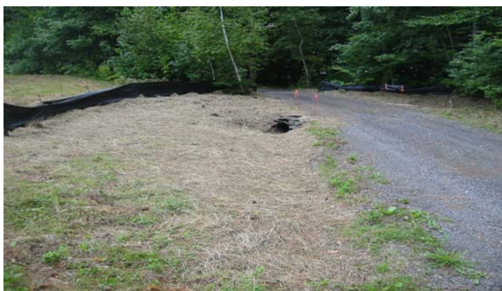
A successful BMP implementation on Dinsmore Lane on Branch Pond New culvert, level-lip spreader and ditch to divert channeled flow away from pond
