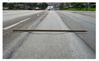
Figure 1. Severity of pavement rutting at an intersection
