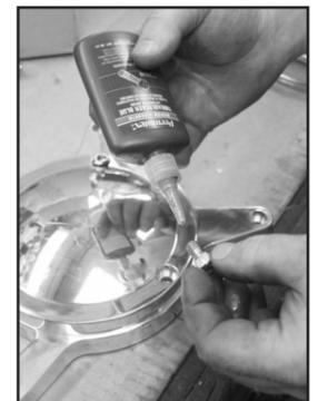
6. Install Outer Cover Caps onto the Outer Cover using Blue Loctite. Torque to 18-22 ft lb. Note the bolt clearance notch location on the motor pulley cap to the outer plate.
